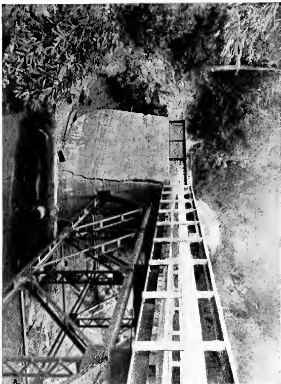
A. Near Watsonville. Concrete pier of bridge shattered. Per J. C. B.
